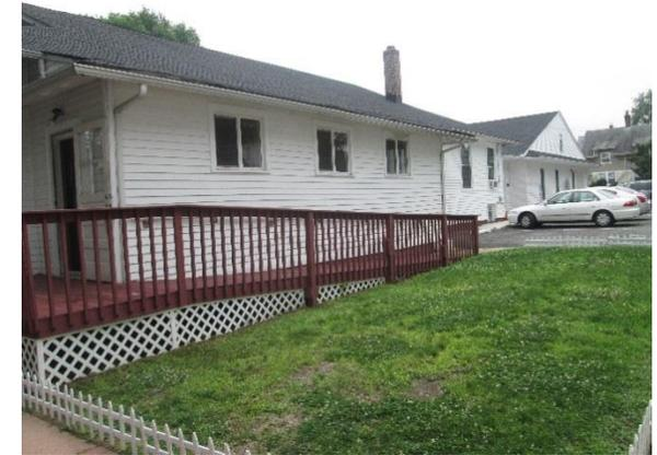
Parking spaces can be replaced with porous asphalt to capture and infiltrate stormwater. Installing rain gardens adjacent to the building can capture, treat, and infiltrate roof runoff. A preliminary soil assessment suggests that more soil testing would be required before determining the soil's suitability for green infrastructure.
