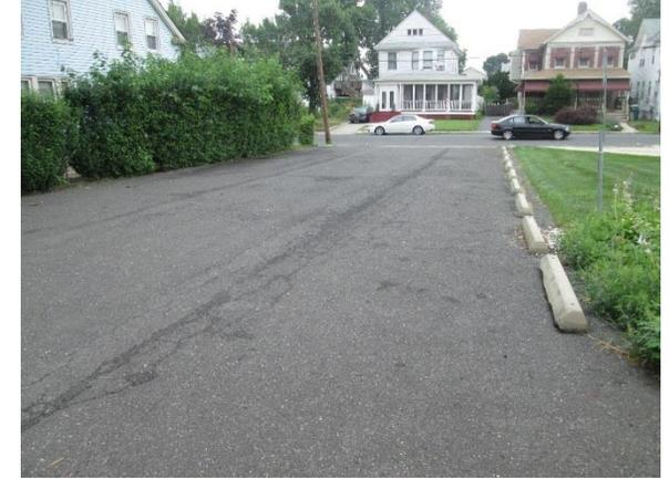
A row of parking spaces can be replaced with porous asphalt to capture and infiltrate stormwater. A preliminary soil assessment suggests that the soils have suitable drainage characteristics for green infrastructure.
