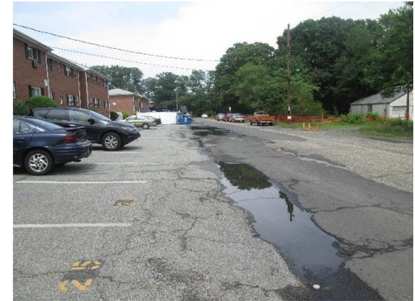
Parking spots can be replaced with porous asphalt to capture and infiltrate stormwater. Multiple rain gardens can be installed throughout the complex adjacent to the buildings to capture, treat, and infiltrate roof runoff. A preliminary soil assessment suggests that the soils have suitable drainage characteristics for green infrastructure.
